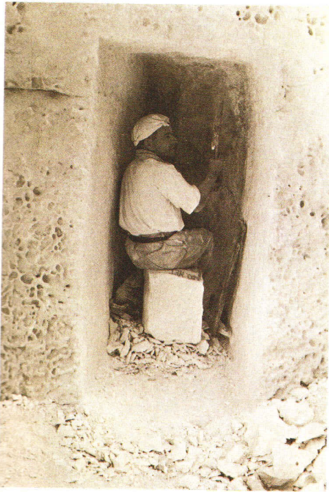
A Maltese civilian cuts a shelter for his family out of the soft limestone.
